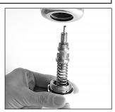
Remove body cap with wrench to service cold water assembly.
