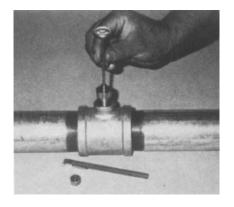
Is instant access to test temperature and/or pressure. Reduce need for permanently installed gauges.
